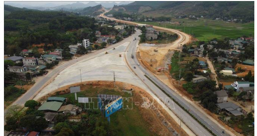
The project under construction
