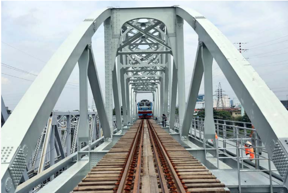
New Binh Loi Bridge
