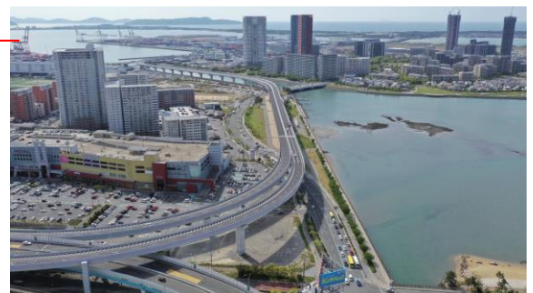
Fukuoka City/ General Subsidy Facilities Improvement Project (Special Sublease Bonds) (Fukuoka Expressway Construction Project)/ Fukuoka Expressway Route 6 (Harbor Road Island City Route 3) Fukuoka City, Fukuoka Pref.
