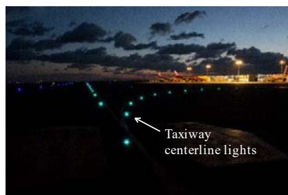
Examples of aviation lights at airports
