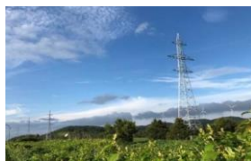
Construction of power grid (image)
