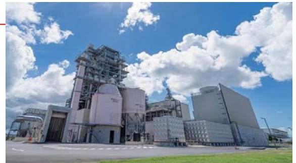
The Okinawa Development Finance Corporation/ Loan to Okinawa Uruma New Energy Corporation (to support installation of Okinawa's largest biomass power plant) / Power Plant / Uruma City, Okinawa Pref.
