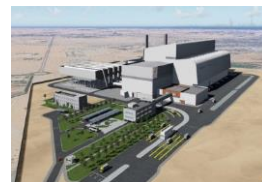
Waste treatment and power generation plant construction and operation (image)
