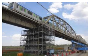
improvement of the earthquake resistance of elevated bridges (image)
