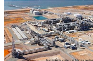
<Natural Gas Liquefaction Business (image)>
