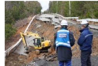
▲ Emergency restoration of roads in cooperation with construction companies.
