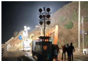
▲ Day and night emergency road restoration with lighting vehicles.
