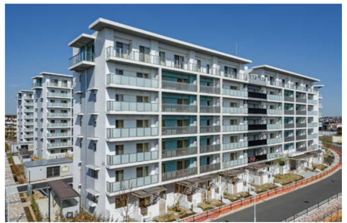
Urban Renaissance Agency / The rental housing program / Rental housing / Chigasaki City, Kanagawa Pref.
