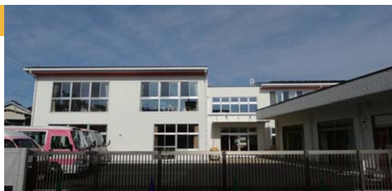
WAM/Welfare loan project/Certified childcare institutions, Ruri Kindergarten/Shizuoka City, Shizuoka
